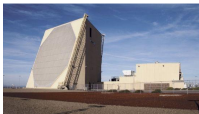
Radar Power supply
