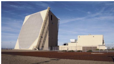
Radar Power supply
